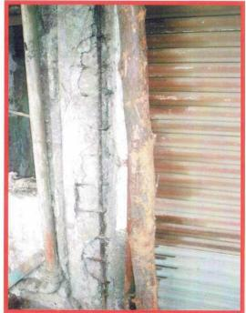
**Photographs Shows: The Core Damaged of Colomn.**
