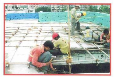
Photographs Shows: Breaking Damage Top Floor Slab by providing supporting platform.
