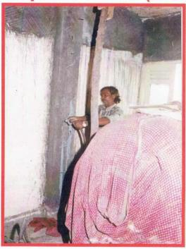
Photographs Shows: Injection grouting to colomn.
