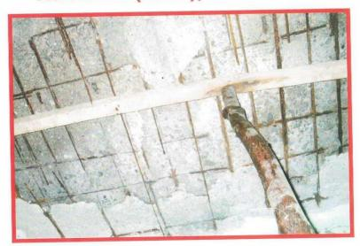
Photographs Shows: Temporary supporting System for Slab
