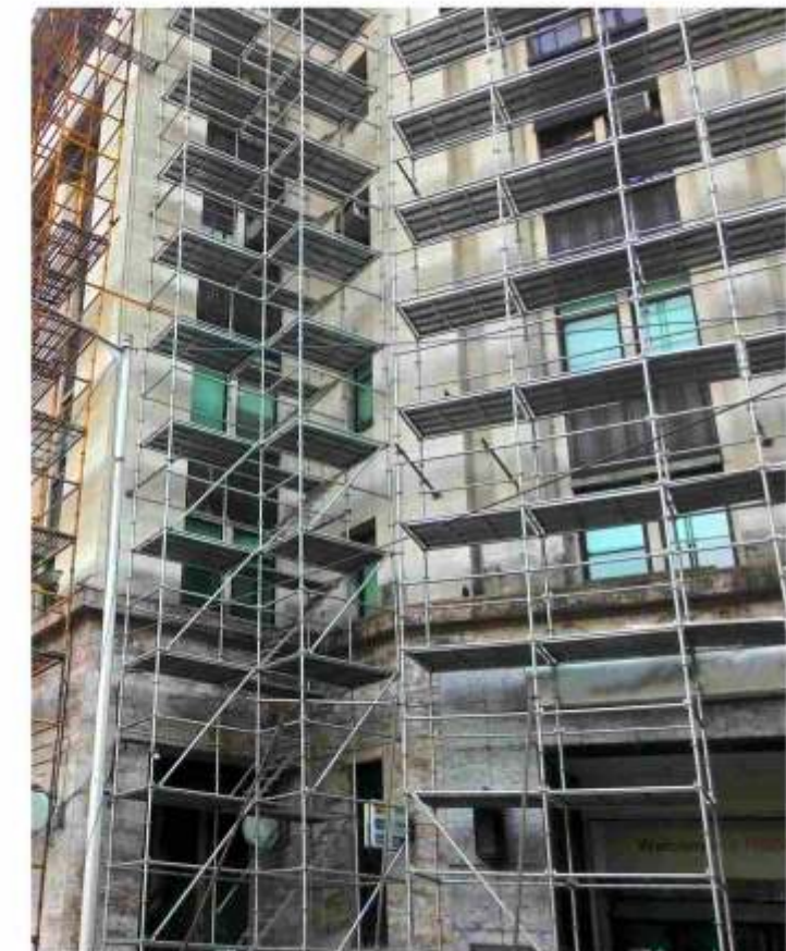
● Modern ring lock system scaffold installed at site
