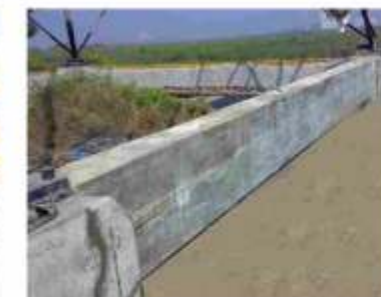
● Section buildup using Microconcrete
