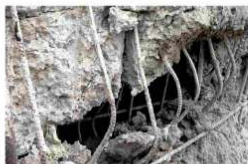
● Crushing of concrete and bending of main reinforcement
