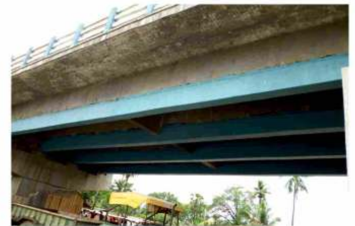
● Application of polyurethane coating
