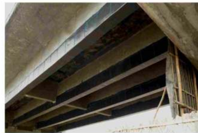
● Application of carbon fiber wrap
