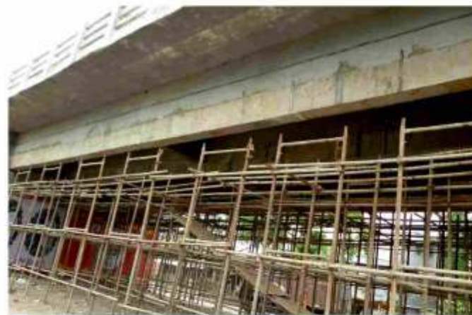
● Rebuilding of section using Microconcrete
