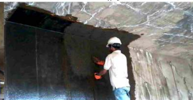
● Carbon fiber wrapping at site
