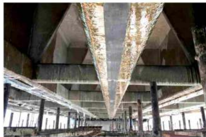
● Post tensioned CFRP Laminate
