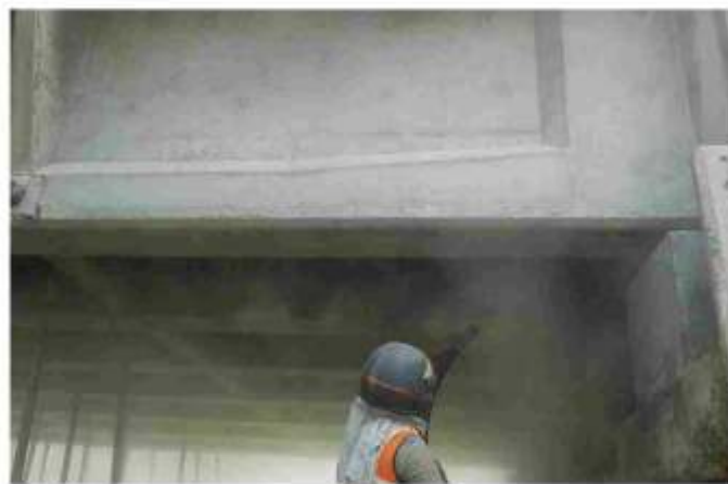
● Cleaning by sand blasting
