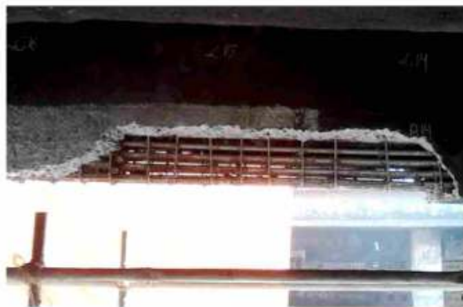
● Reinforcement congestion at the bottom leading to hollow section
