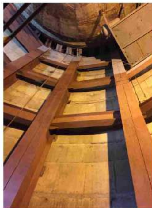
● Hopper supported with additional MS frame
