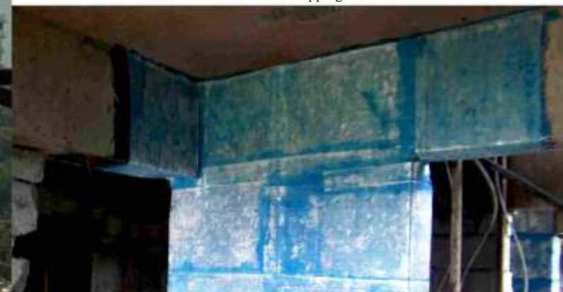
● Glass fiber wrapping at site
