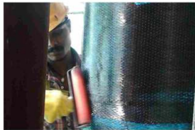
● Fiber wrapping of column
