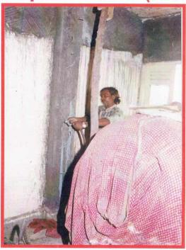
Photographs Shows: Injection grouting to colomn.
