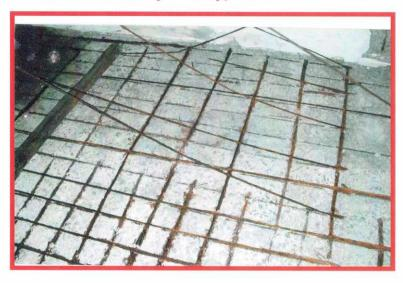
Photographs Shows : Damaged condition of Slab.
