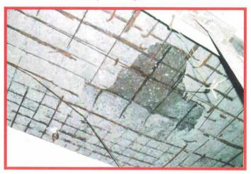
Photographs Shows: Debounded bottom concrete at Bars Corroded.
