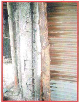
**Photographs Shows : The Core Damaged of Colomn.**
