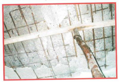
Photographs Shows: Temporary supporting System for Slab
